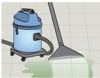
Remove slurry with wet suction machine or mop.
